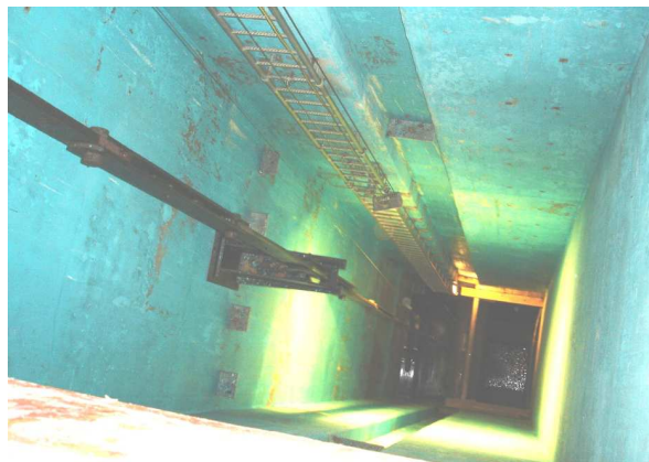
Figure 1: View into the duct of the slide gate chain
