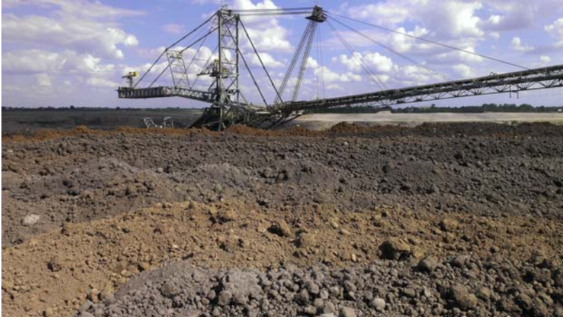
Picture 11.1 Backfilling of an open-pit mine.
