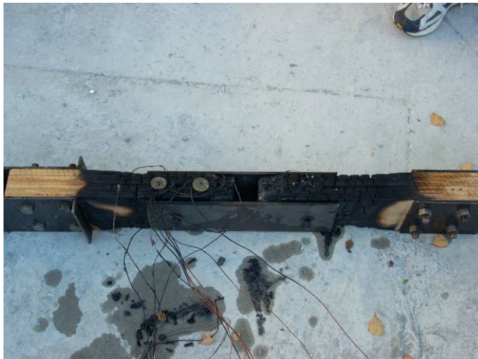
Sws connection with one bolt after a fire test
