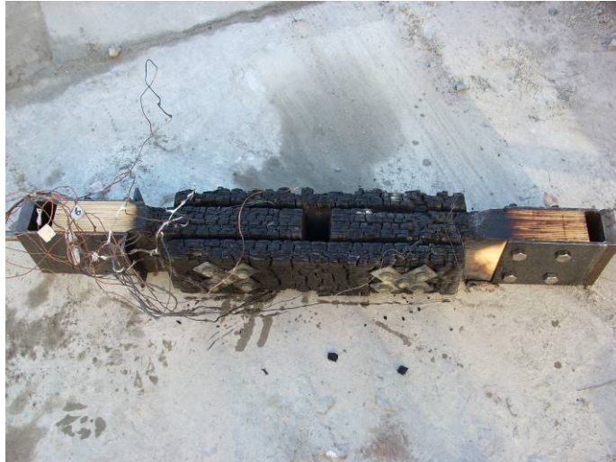
www connection with 5 bolts after a fire test
