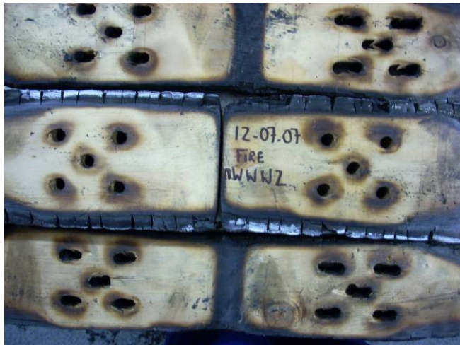
www connection with 5 bolts after a fire test. The timber on the side members is crushed so this is mode g.
